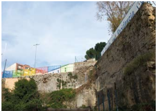
↑ Part of the wall in the western area of the city. (David Grau)
